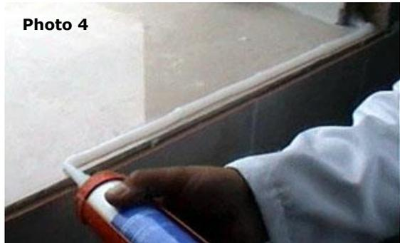
After the frame installation, apply an additional continuous silicone bead on all the perimeter on 3 sides of the frame.
